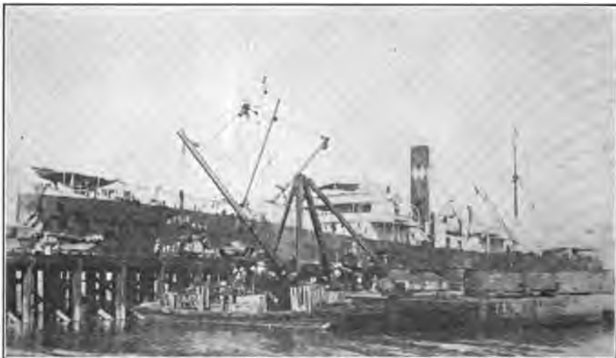
FIG. 152.—Unloading heavy machinery on to lighters and to wharf in an isolated harbor in the Philippine Islands. The steamship's "heavy lift" boom (see p. 375) is clearly shown.
